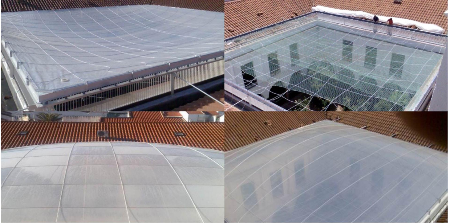
ETFE membrane (15x15 cm air bag on 250 microns EFTE with wired mesh)
